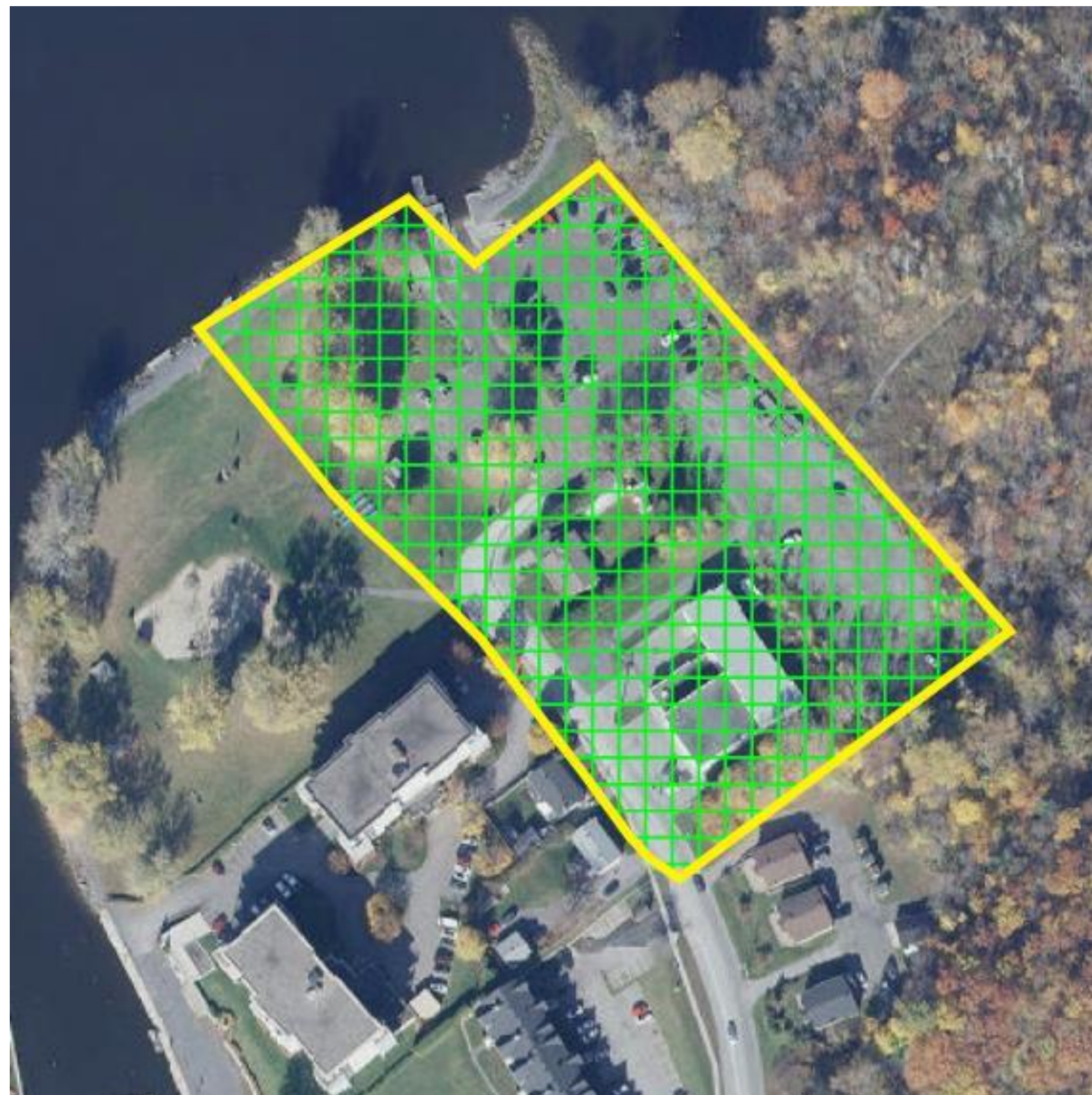
Rockland WTP (147 Edwards St., Rockland, ON)
