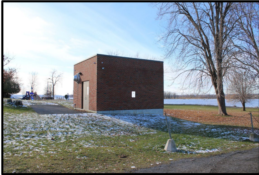
Figure 3. Rockland WTP Low Lift Pump Station. Matrix Heritage, Nov 19, 2025.
