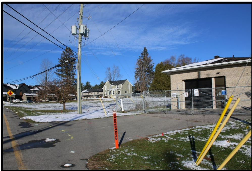
Figure 33. View looking north-east of Caron BPS. Matrix Heritage, Nov 19, 2025.
