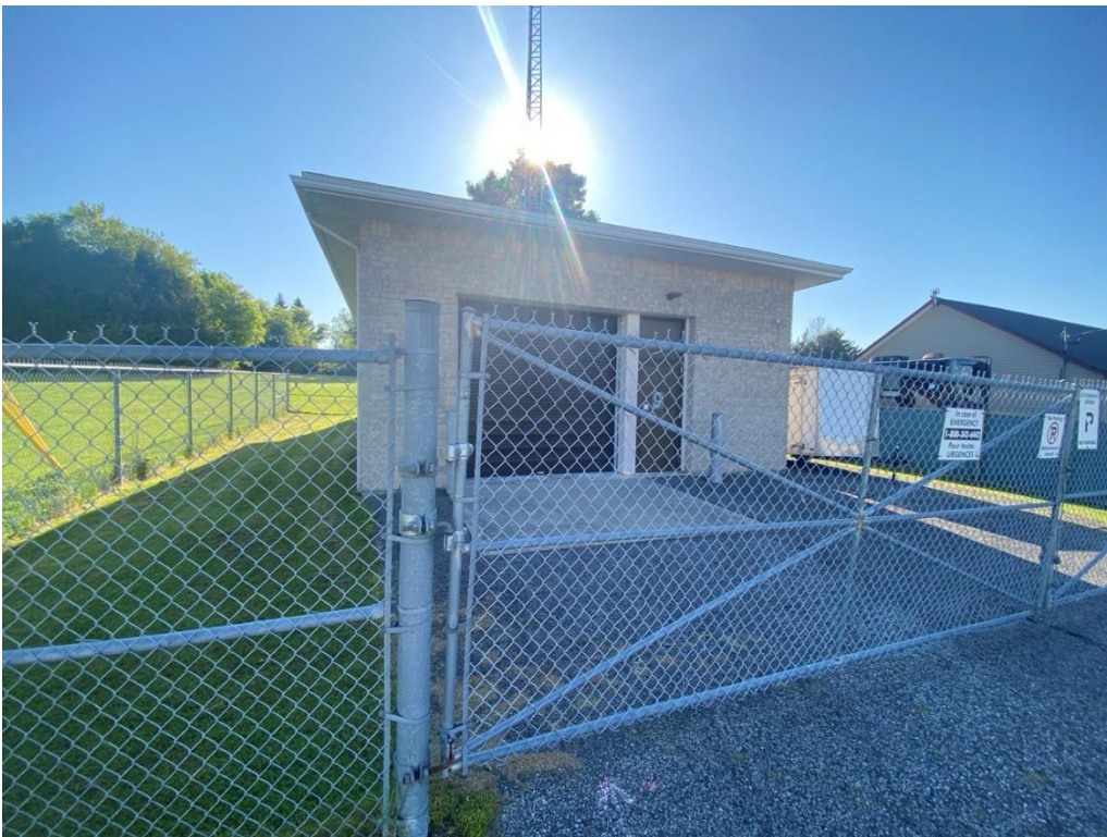
Photo 6. Photo taken facing east of the Caron Booster Station.
