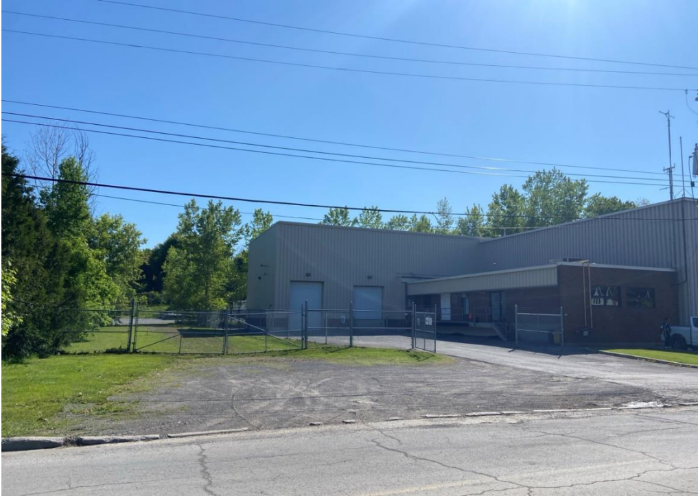
Photo 1. Photo taken facing east, from Edwards Street, of the existing WTP building, located within the Industrial Zone.
