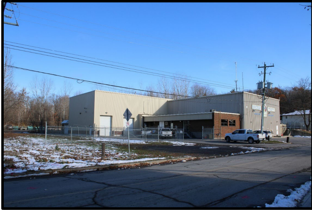
Figure 1. Rockland Water Treatment Plant located at 147 Edwards St. Matrix Heritage, Nov 19, 2025.
