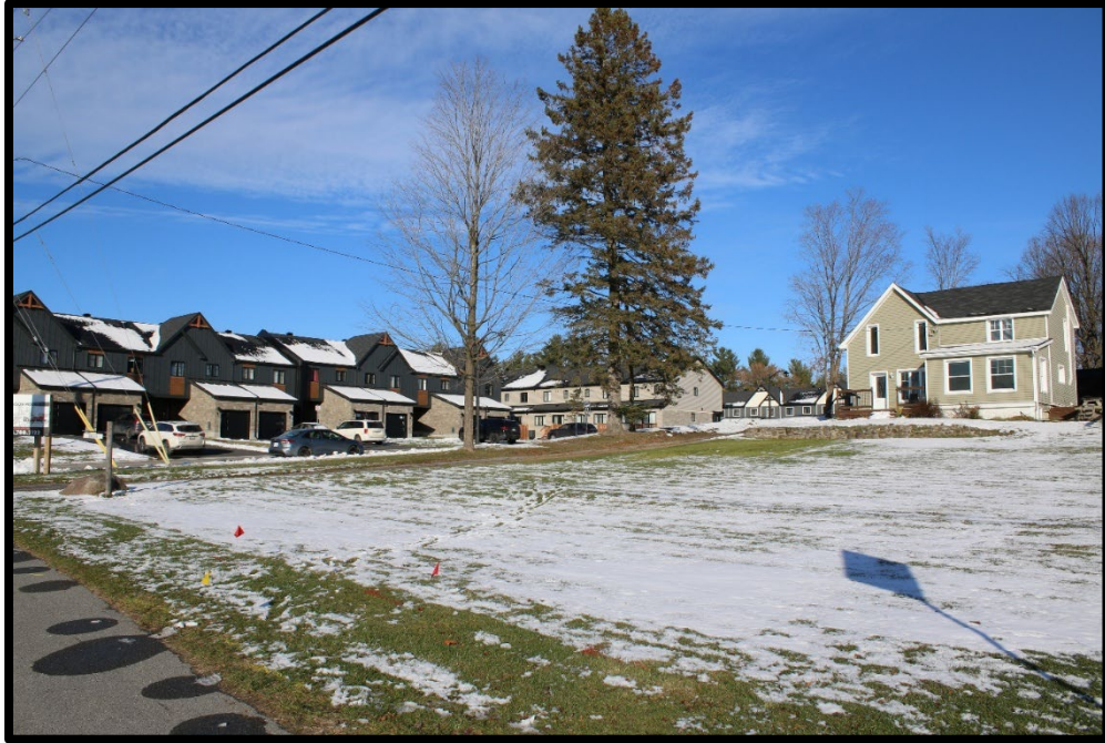
Figure 38. 1433 Caron St. and new Darquise St. subdivision development, north of the Caron BPS. Matrix Heritage, Nov 19, 2025.
