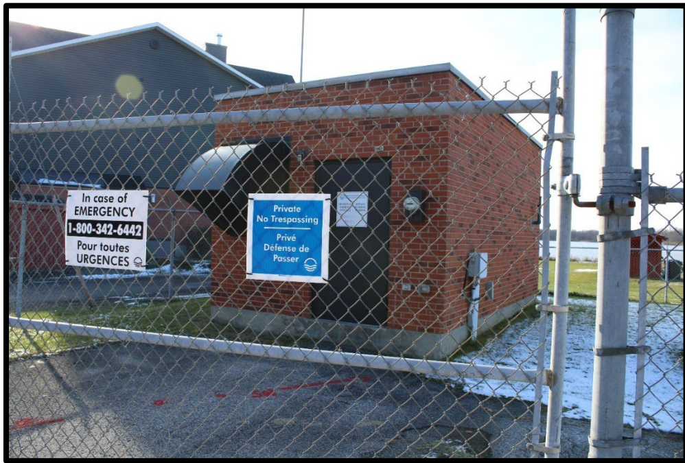
Figure 29. Sewage Pumping Station, Edwards St. Matrix Heritage, Nov 19, 2025.
