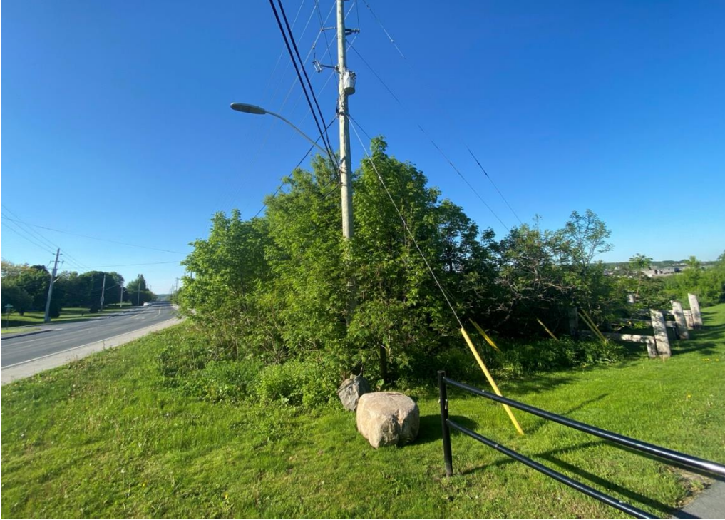
Photo 9. Photo taken facing south of the Parkland community located across the street from the Caron Booster Station.
