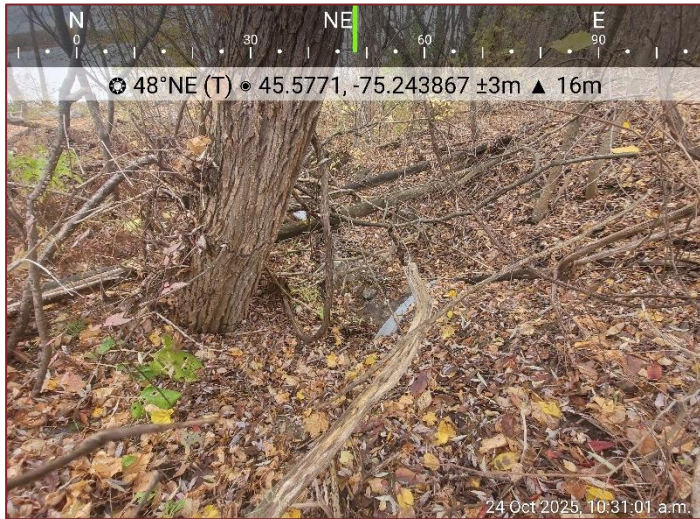
Site Photograph 11 – Unnamed Watercourse Culvert Outlet
