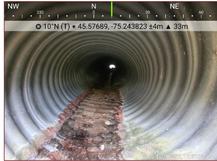
Site Photograph 10 – Unnamed Watercourse Culvert Inlet
