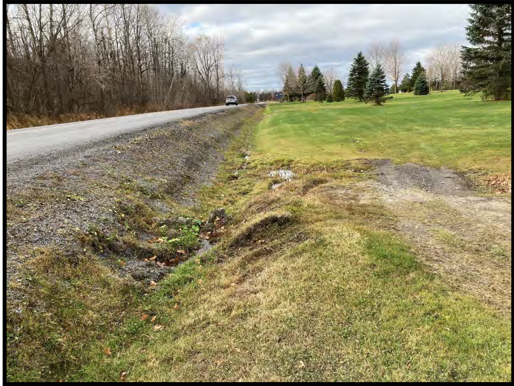
Figure 51: Gravel shoulder and ditch, gravel fill. (MH1125-D189)
