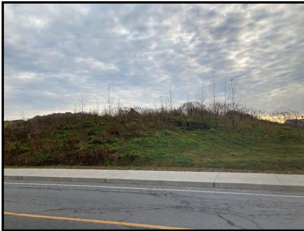
Figure 40: Sidewalk, ditch, and banked soil from new subdivision. (MH1125-D070)
