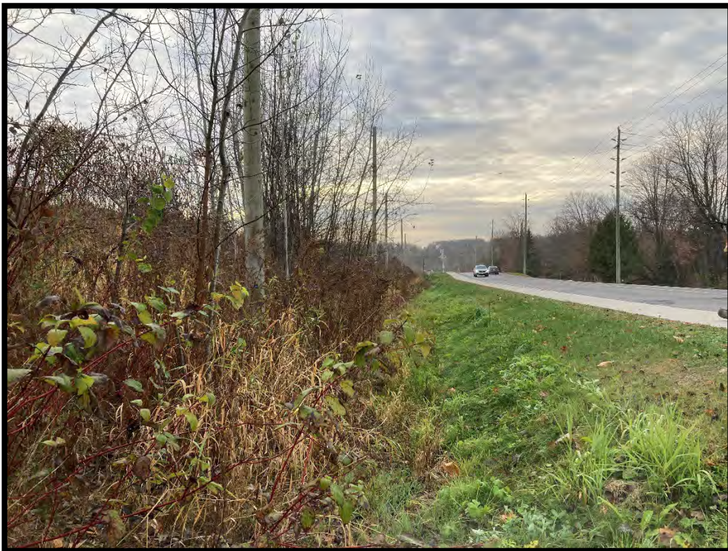
Figure 38: Steep ditch and banked soil. (MH1125-D051)
