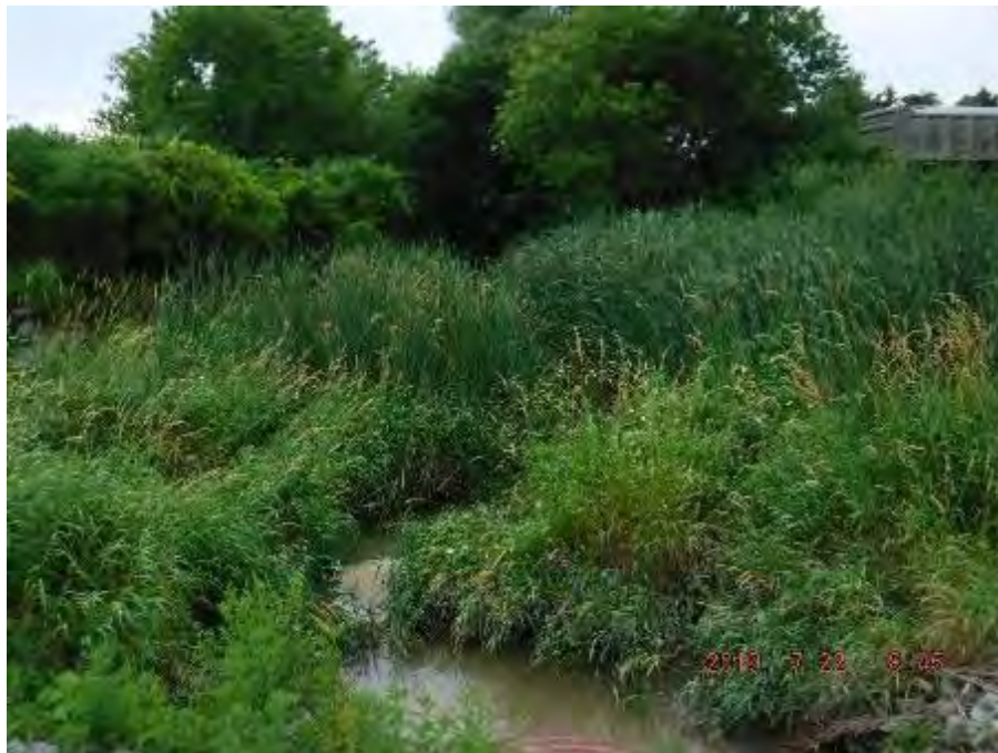
Photo 26 : Station 2 looking upstream from the downstream end (July 22, 2019)
