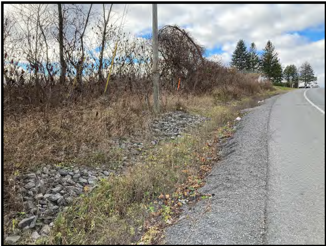
Figure 4: Steep slope with ditch and large stone gravel. (MH1125-D151)
