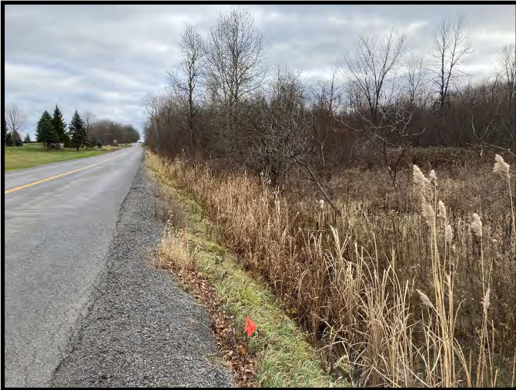
Figure 54: Ditch on southern side with gravel shoulder, marshy conditions, buried utilities. (MH1125-D220)
