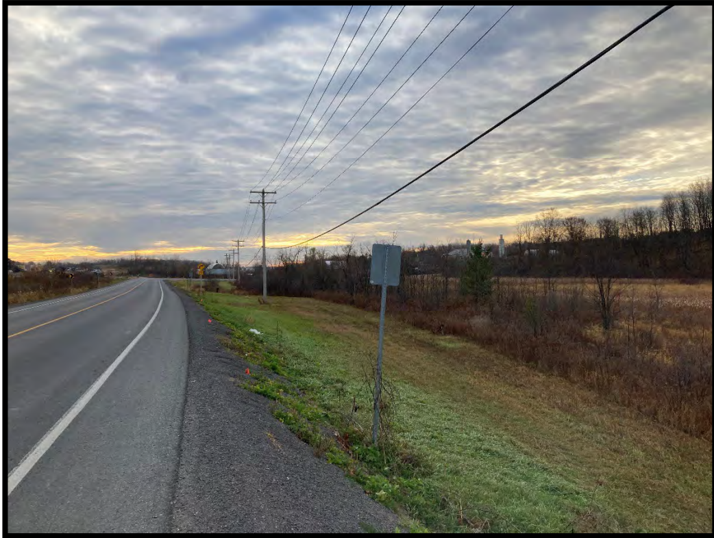
Figure 43: Steep ditch to large marshland, buried utilities. (MH1125-D093)
