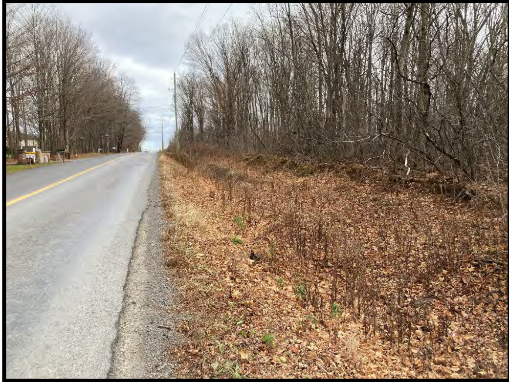
Figure 11: Ditch with banked soil on southern side. (MH1125-D233)
