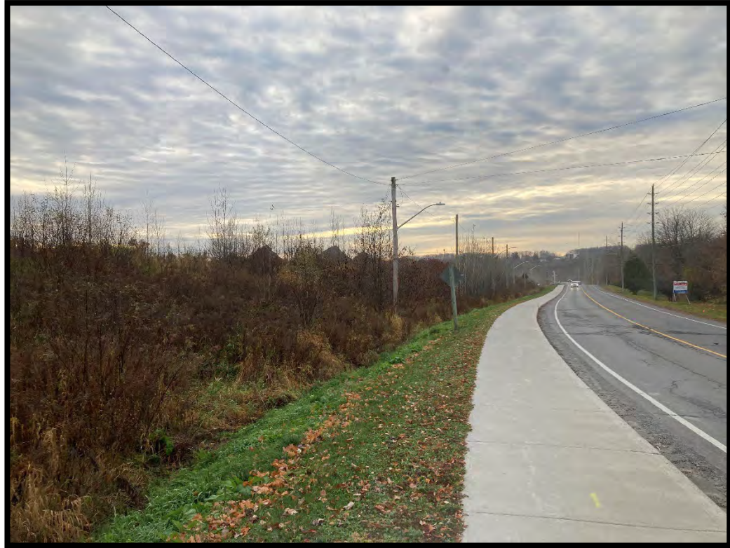
Figure 35: Concrete sidewalk with banked soil and buried utilities. (MH1125-D044)
