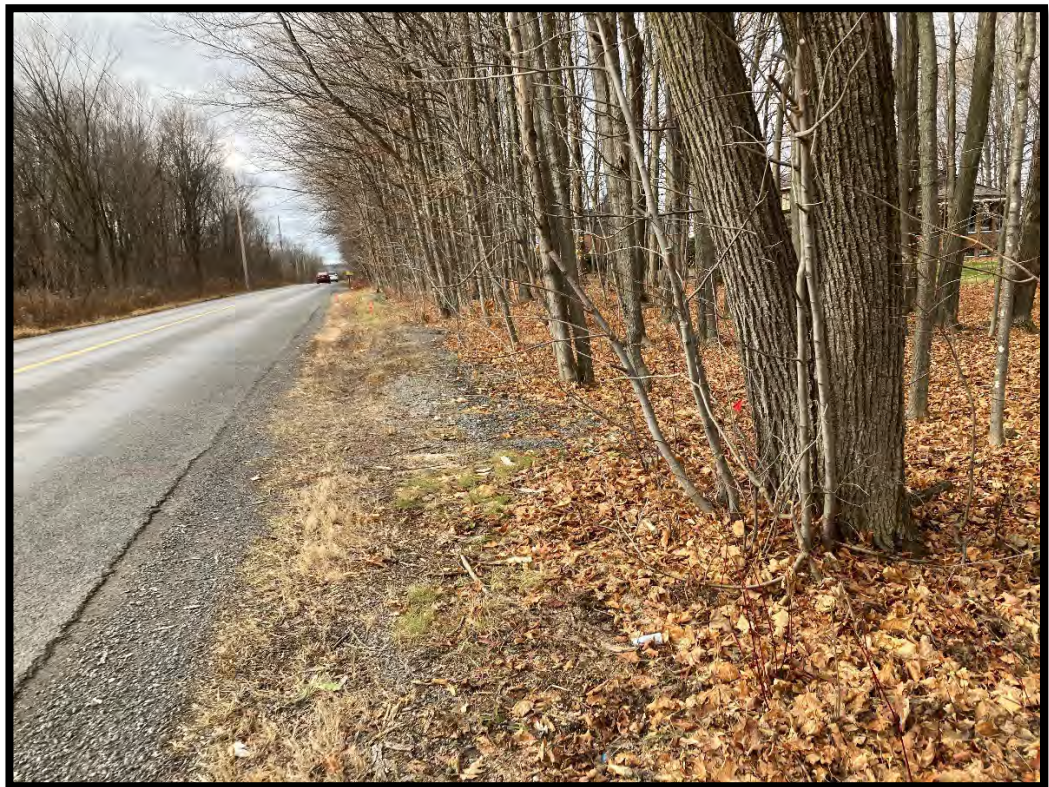
Figure 8: Gravel shoulder by houses with buried utilities, northern side. (MH1125-D171)
