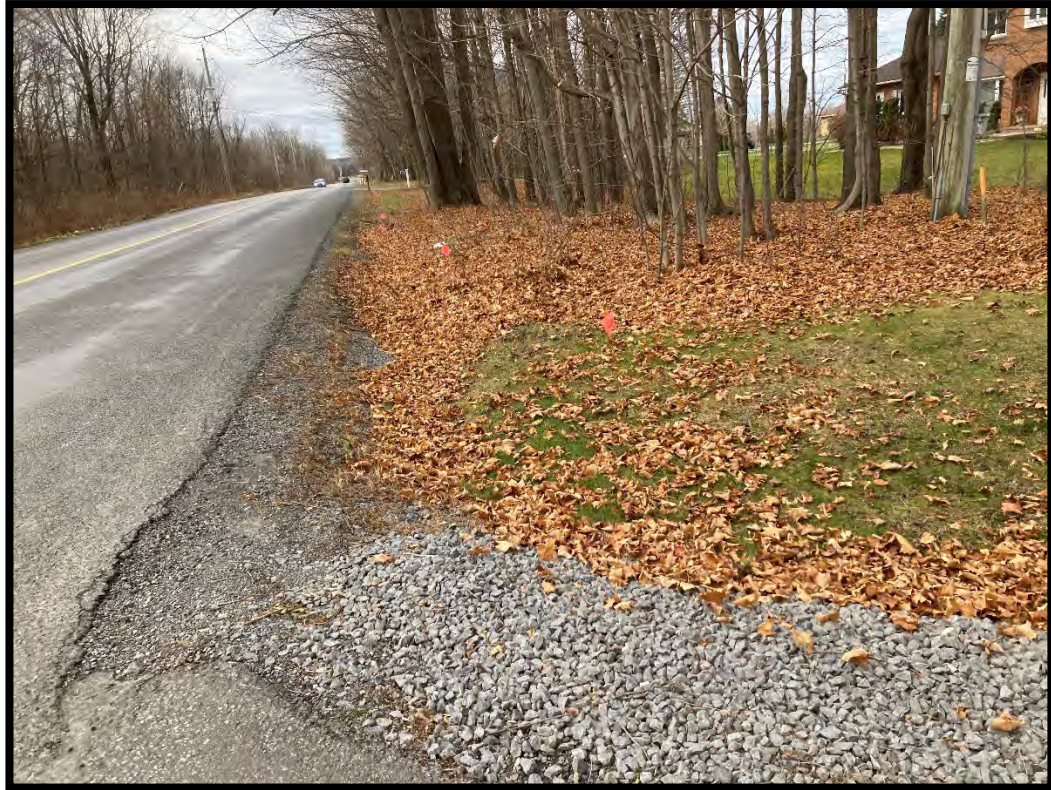
Figure 15: Gravel should and ditches, showing buried utility lines. (MH1125-D175)
