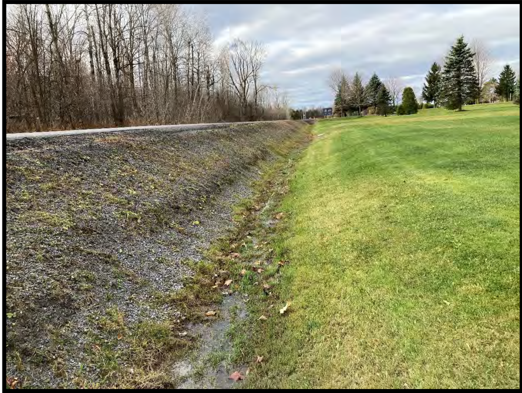
Figure 5: Ditch with gravel shoulder. (MH1125-D190)
