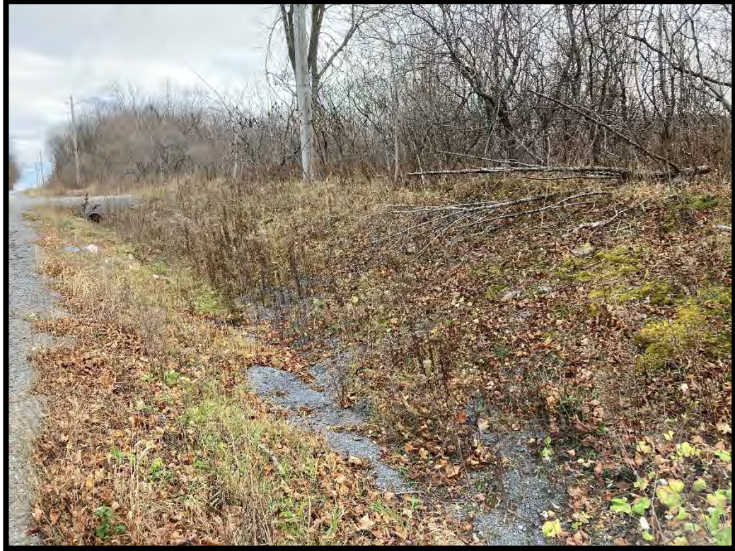
Figure 55: Ditch with gravel shoulder and fill bank visible. (MH1125-D227)
