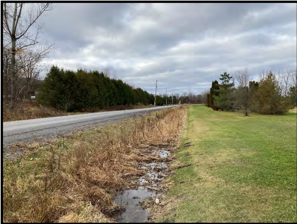
Figure 6: Ditch with gravel shoulder. (MH1125-D198)
